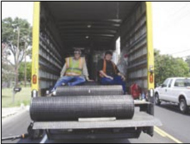
GlasGrid® arrives in 5ft (60 inches) wide rolls so it stays dry.
