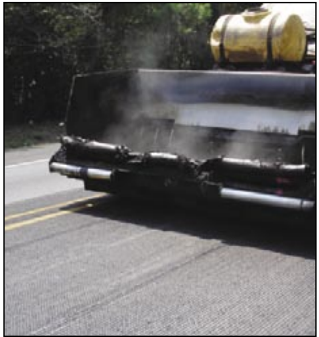
GlasGrid® remains flat and wrinkle-free during paving. Use of a tack coat should be dictated by project conditions, application and/or specifications.
