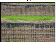
Grade Separation Solution utilizing Tensar Uniaxial (UX) and Biaxial (BX) geogrid, galvanized wire basket forms, woven geotextile and permanent erosion control matting
