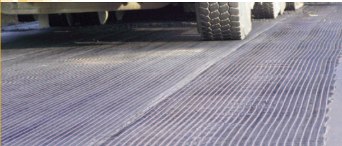
The GlasGrid® System is able to withstand construction equipment trafficking before being overlaid.
