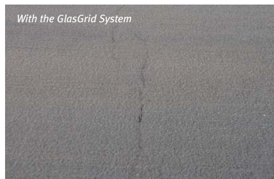
Pavement surface condition following 11 years of post-rehabilitation service.
